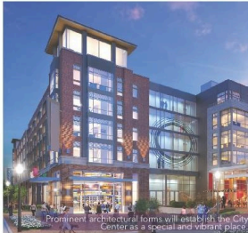
Prominent architectural forms will establish the City Center as a special and vibrant place.
